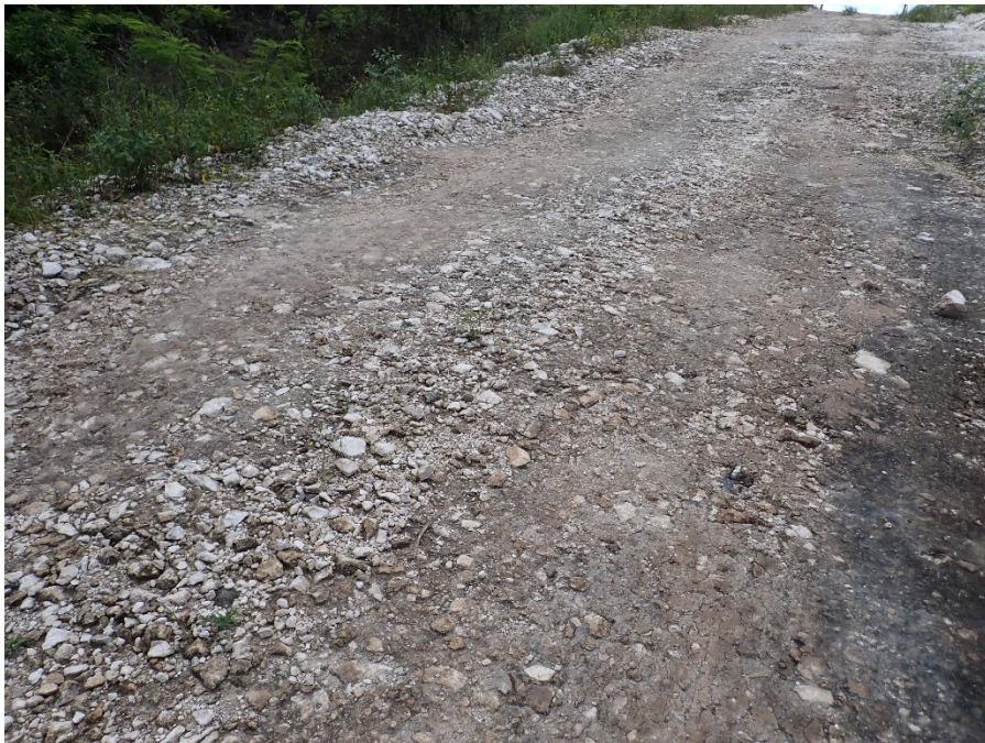
Photo 7: Bare Road/Paved Surface.
